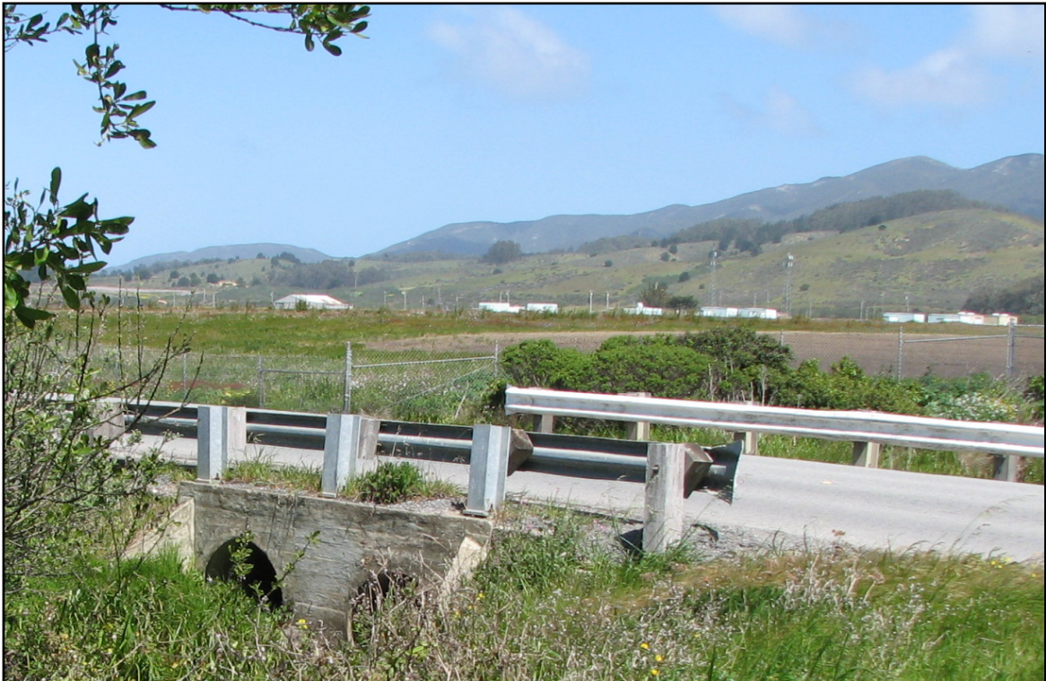
Surface water drainage culverts on site.
